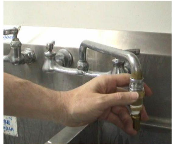
Connect Auto-Fill Water Supply Hose to machine and faucet
